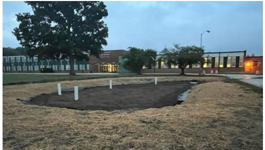
The Surrattsville High School project was completed in August of 2022. Devices installed include a micro-bioretention and Nyoplast drain. The MMBR device will be treating 12,340 square feet of impervious area with a maximum drainage area of about 20,000 square feet. NARDI was proud to be part of another Mentor Protégé project (MPP) with the Clean Water Partnership. The project was completed by new MPP member AC Reliable Construction, Inc.
